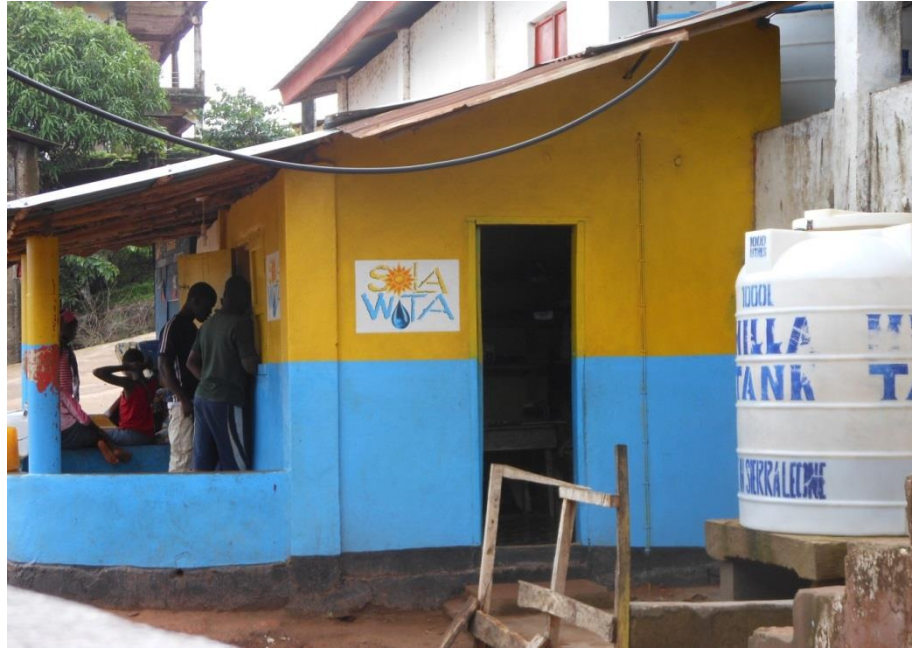
Figure 2: The Kassirie CCS, used for the production and sale of SolaWata and mobile phone charging
